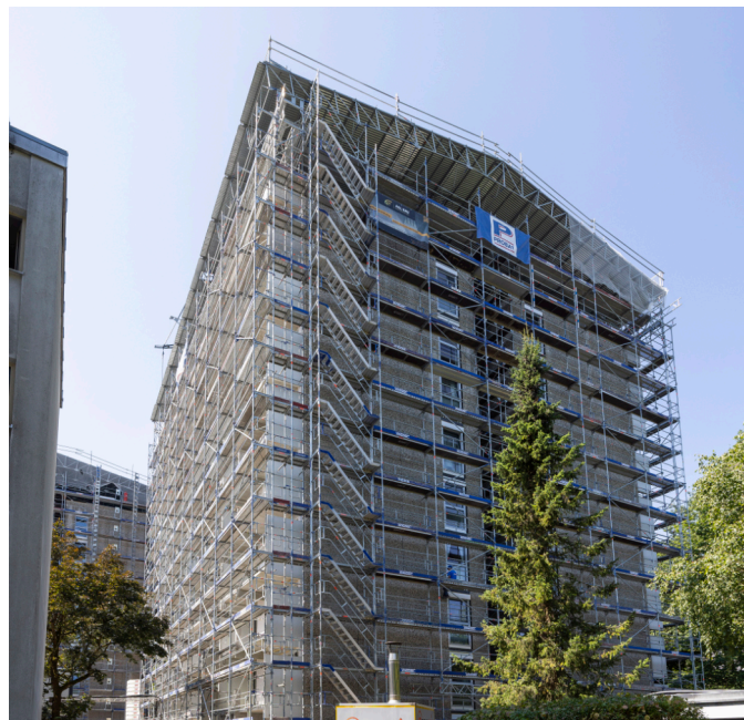
Renovation work on existing buildings in the neighbourhood
