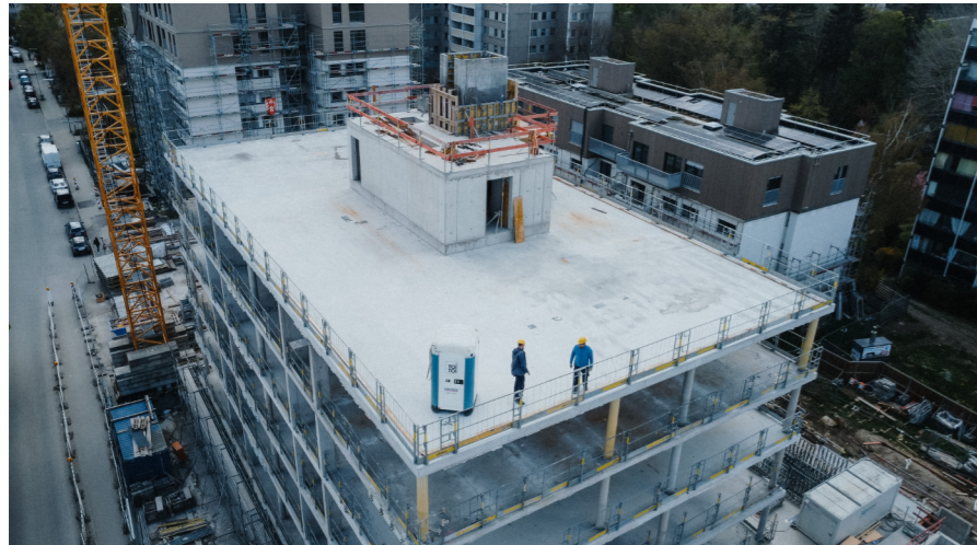
Construction site at the future neighbourhood square in the summer of 2026
