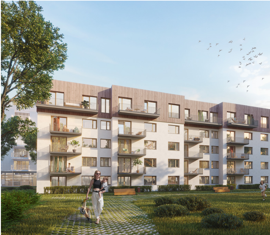
Completed addition of storeys to Haus Marwees (Appenzeller Str. 115-117)
